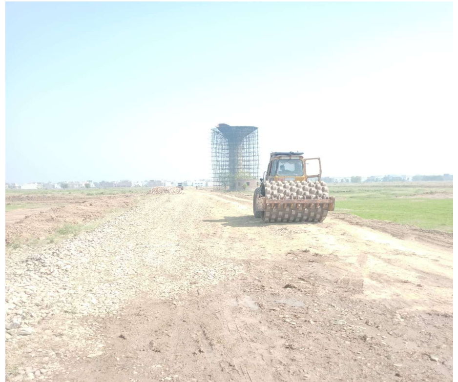
Compaction of sub base at road no.16
