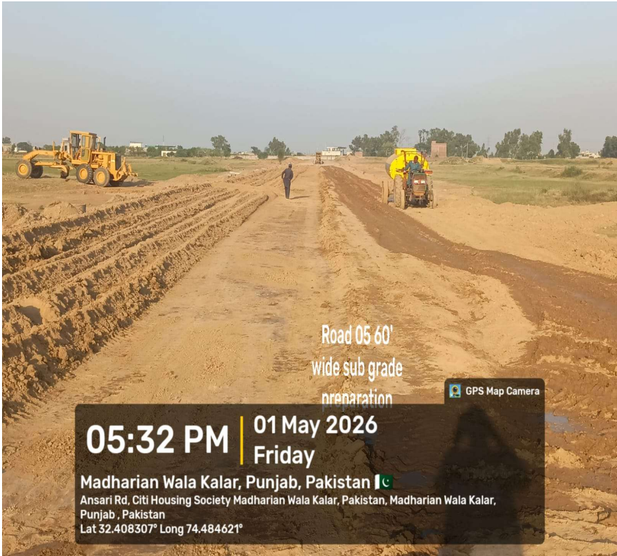
Preparation of sub grade top at Road no.5 (60 ft wide)
