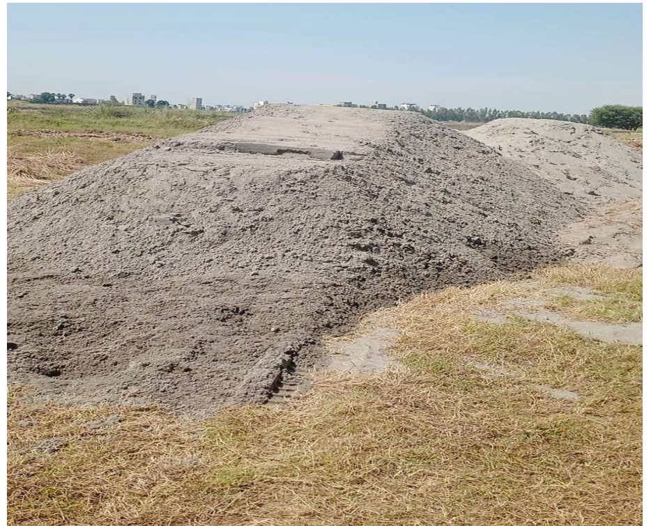
Dumping sand for water supply line (under and around)
