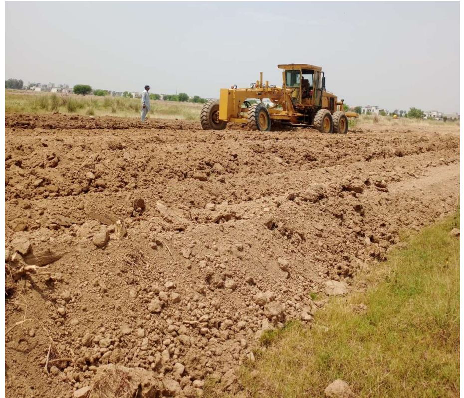
Laying of sub base at road no. 14 (60 ft wide)
