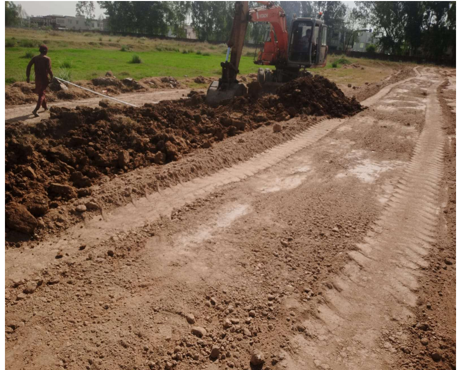
Excavation for Water Supply line 4" dia
