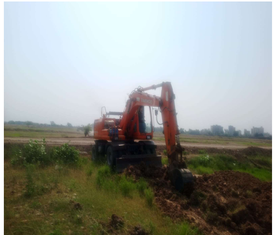
Excavation for water supply line
