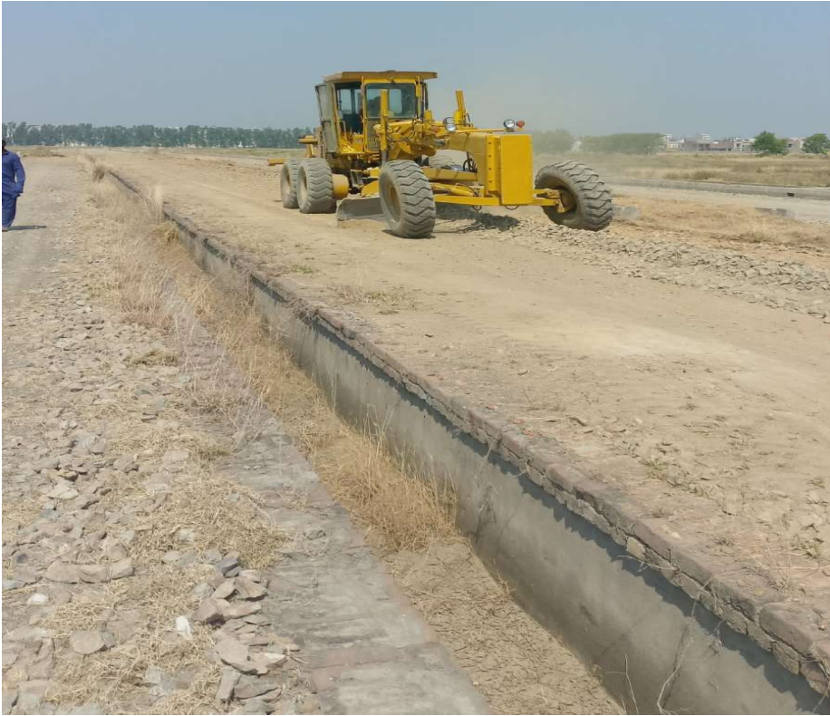
Preparation of sub base at main boulevard
